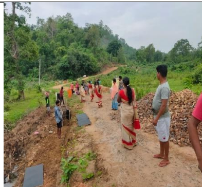
Asset verification at Rayagada district
