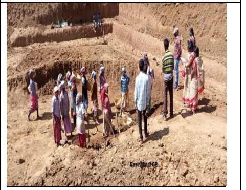
Beneficiaries verification as per MR at worksite in Kandhamal district
